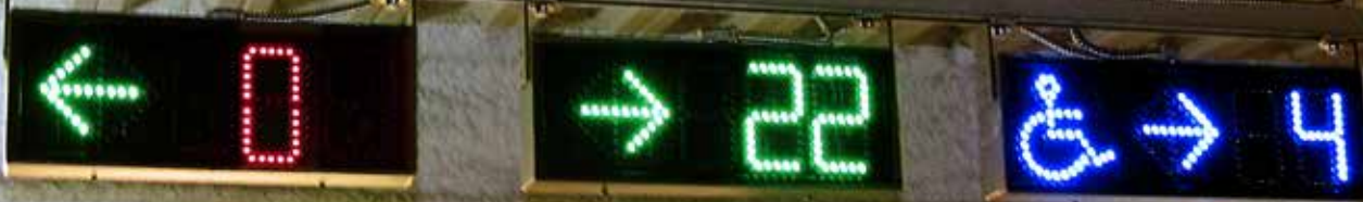
Parking Garage Cosmopolitan Casino - Las Vegas, NV Level by Level - End of Aisle Space Available Signs
